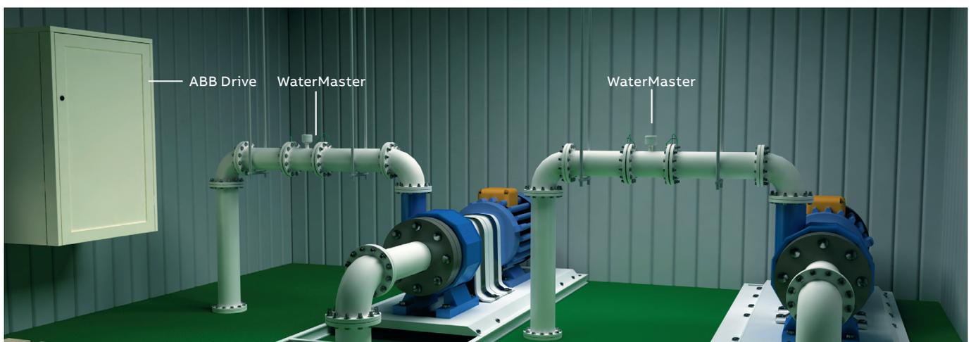
Electromagnetic flowmeters such as ABB's WaterMaster offer long term accuracy and high performance in pumping station applications.
